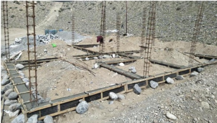
Foundation construction of health center
