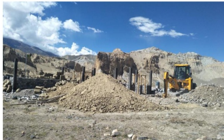
Pillar standing and digging septic tank
