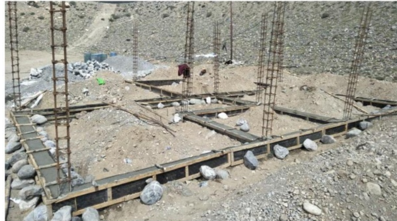
Foundation construction of health center
