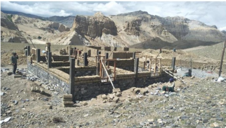
Clay Mud Brick for house wall construction
